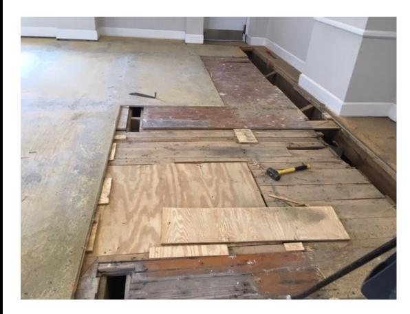
From the start of removing the flooring, we realized that we may be dealing with some significant issues as this photo indicates. Underneath the plywood floor, was a patchwork of scrap wood that was used to "level" the floor.
