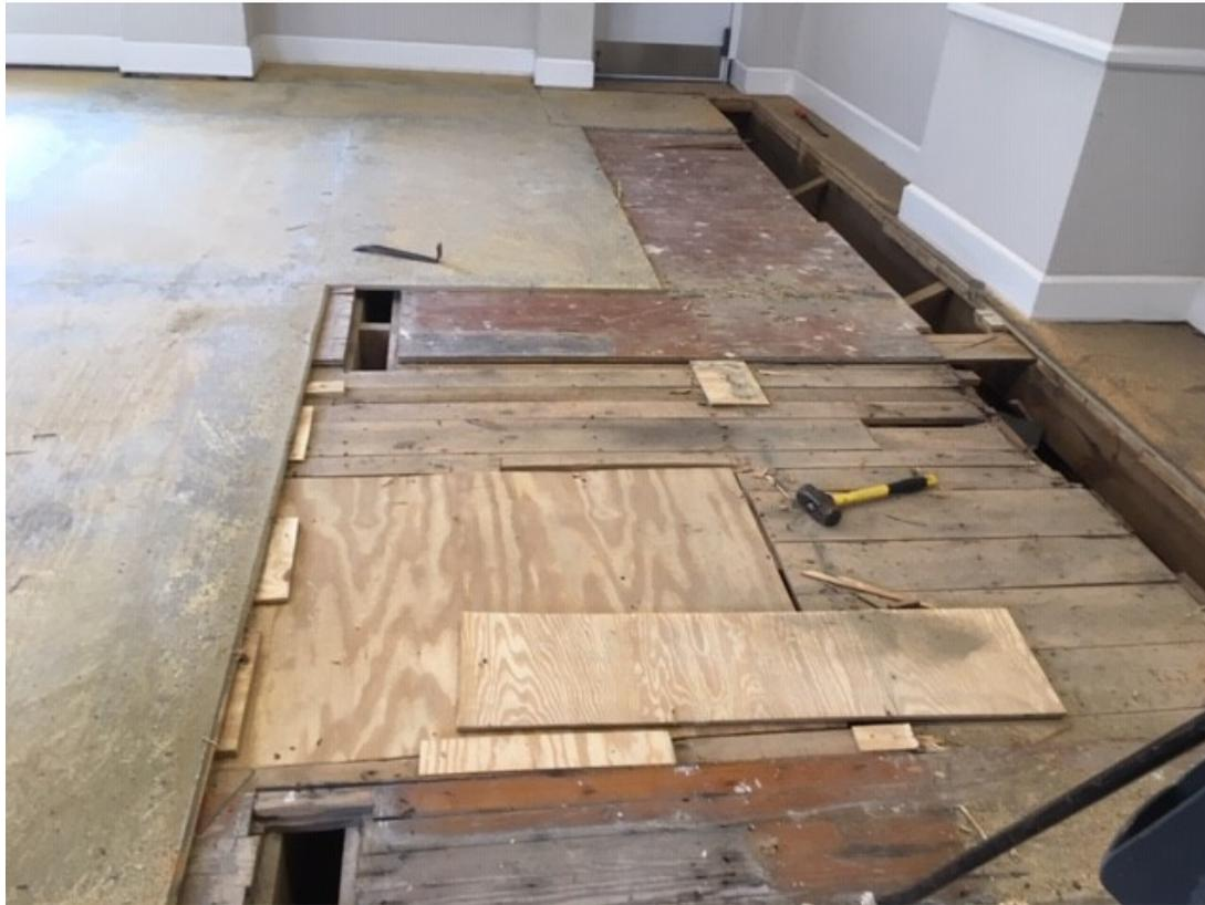
From the start of removing the flooring, we realized that we may be dealing with some significant issues as this photo indicates. Underneath the plywood floor, was a patchwork of scrap wood that was used to “level” the floor.
