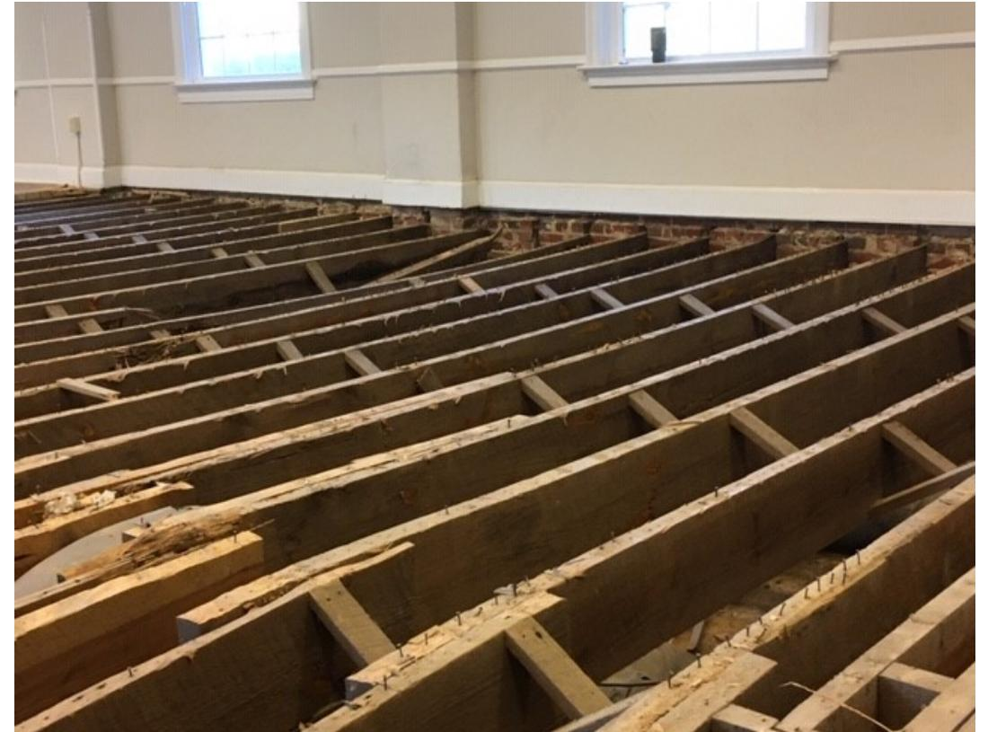
mite damage to the extent they would crumble in your hand or break into pieces when they were lifted.
